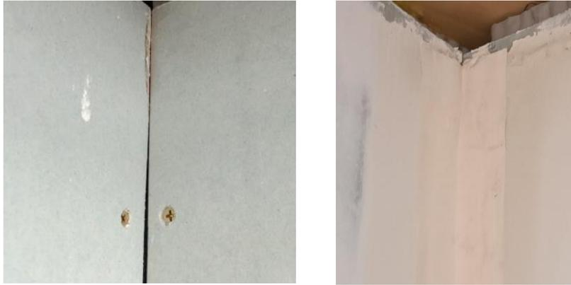
Figure 6: Examples of damage at DS1. Minor movement in linings may cause cracking and/or screw pull through.
