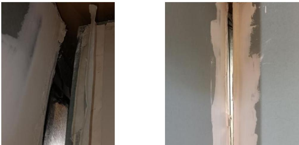
Figure 8: Damage at DS3. Failure of stud connections at corners and damage to framing.
