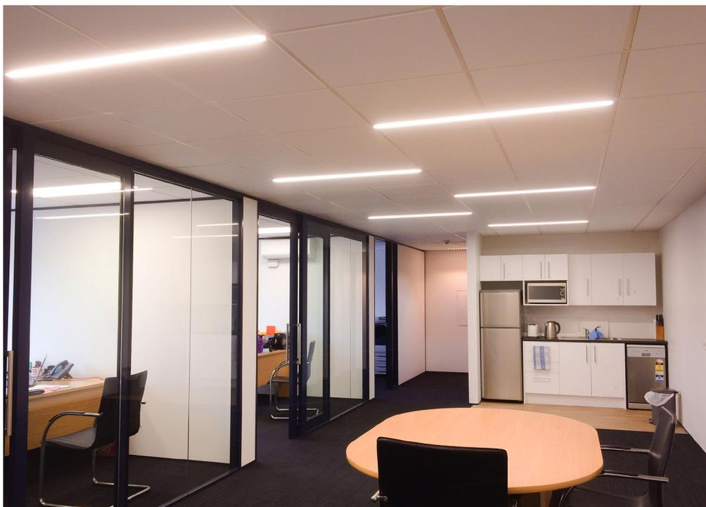
Please Note: Gridlux is installed as part of the ceiling, and should be tendered as part of the ceiling contract. Installation will need to be coordinated with the electrical contractor for power points in the plenum.
