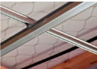
The T&R Screw Fix System is a flexible, high quality, cold formed steel, direct fix or fully suspended grid system, specifically designed for screw fixing sheet linings to form flat monolithic ceilings, bulkheads and strapping.
